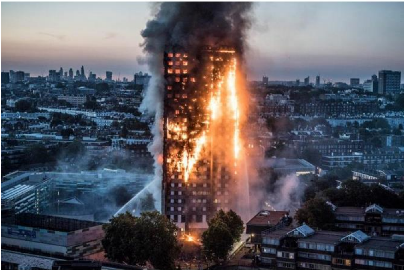
Incendio Grenfell Tower Londra_ ©telegraphcouk
